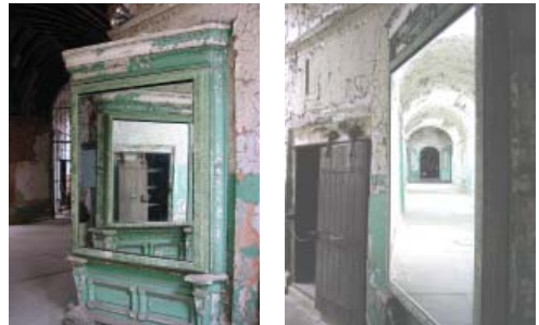
03 | Above: Corridor at cell block 9 (1890's) from Eastern State Penitentiary: Crucible of Good Intentions ; Norman Johnston. Below: Mirrors added before 1900 with cell blocks 8 and 9 were placed at an angle to reflect views so that guards could visually patrol new wings..
